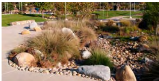
Bio-swale disguised as a dry stream bed at Briarcrest Park in La Mesa.
